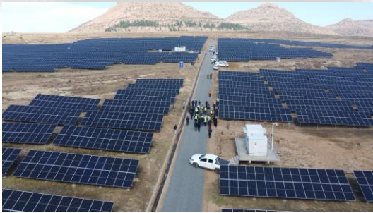
30MW Solar Plant commissioned 2023 - LEGCO
